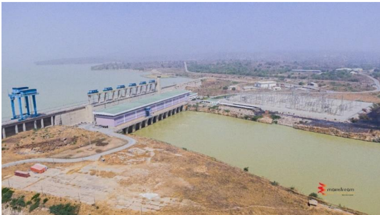
Figure 5: Ariel View of Jebba Hydro power plant
