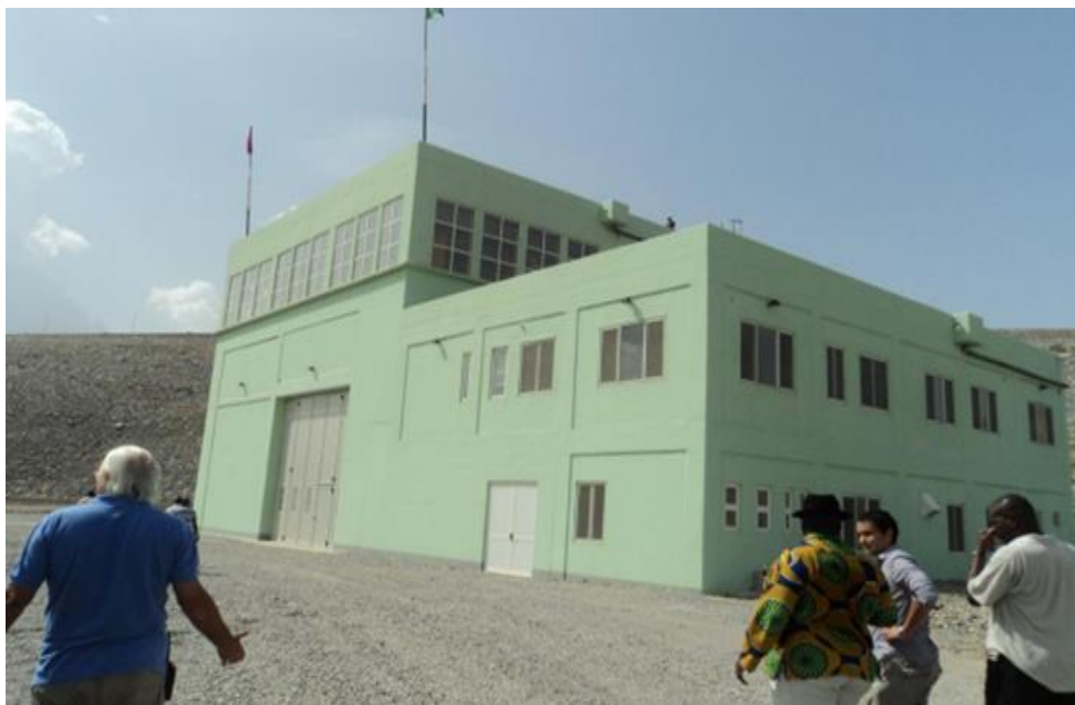
Figure 2: Gurara Power House
