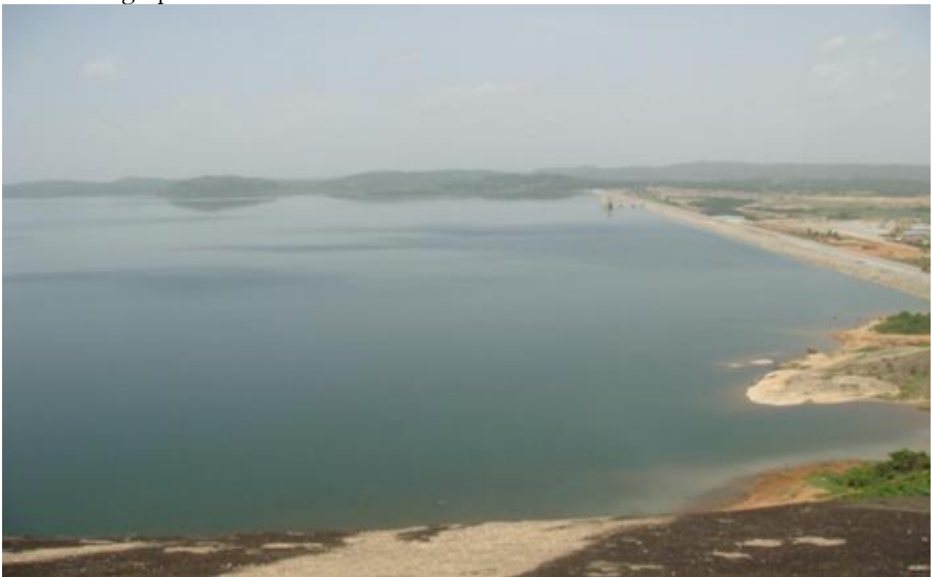
Figure 1 Aerial view of Gurara Dam
