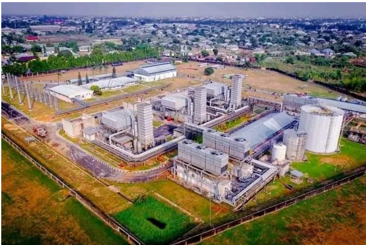
Geometric Power Project in Aba, Abia state - Source: Businessday Newspapers
